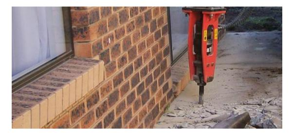
Sandvik's BR111, BR222 and BR333 models combine simplicity and cost-effectiveness with a class-leading power to weight ratio that is optimised for demolition and recycling applications. The three models match carriers in the 0.8 to 4.0 ton (1800-8800 lb) range, and all three breakers utilize a streamlined and lightweight design that sets a new standard in low weight and high power.
