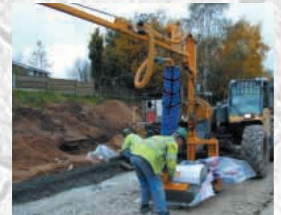
Lifting splayed kerbs
