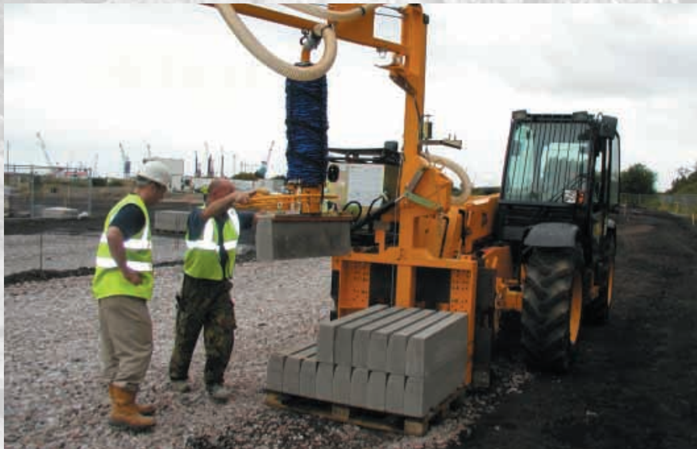
"This machine takes the hard work out of kerb laying."
